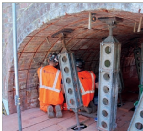
➔ Arch barrel reprofiling
